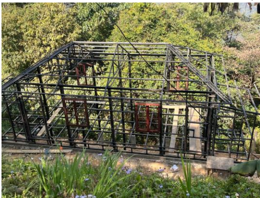
Teacher quarter under construction
